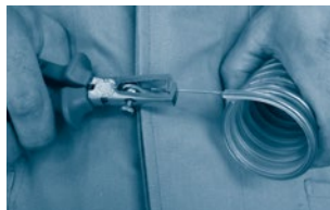
Step 2: Remove plastic from around the wire with a wire stripper...
